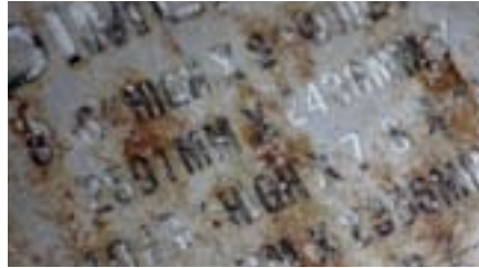
Road Salt Corrosion Damage
